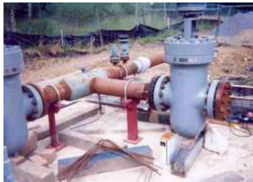
60km Jet Fuel Cross Country Pipeline Upgrade From Class 300 to 600 South of England, UK
